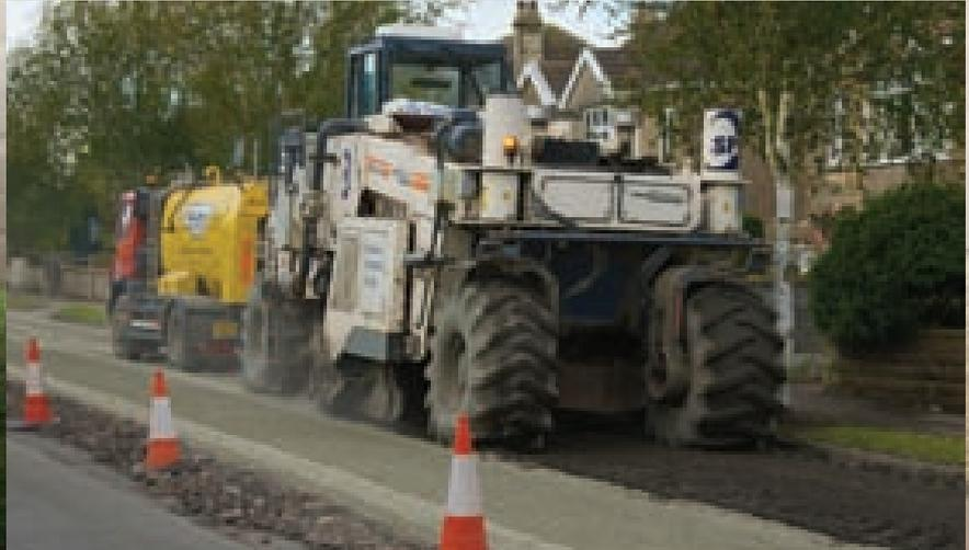
A blend of cement and pulverised fuel ash was spread as a blanket across the rotovated material to strengthen in-situ the tar bound road.
