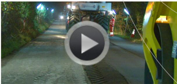
One of the busiest roads in Somerset the A39 Bath Road links Bridgewater and Glastonbury with junction 23 of the M5. Suffering from extensive edge failure, the original scheme required a 6 week closure of the carriageway to carry out the required excavation and re-instatement along this stretch. But to undertake such an extensive closure on such an important road within the network would have been a major headache for the local authority and the people who use the route continuously.
