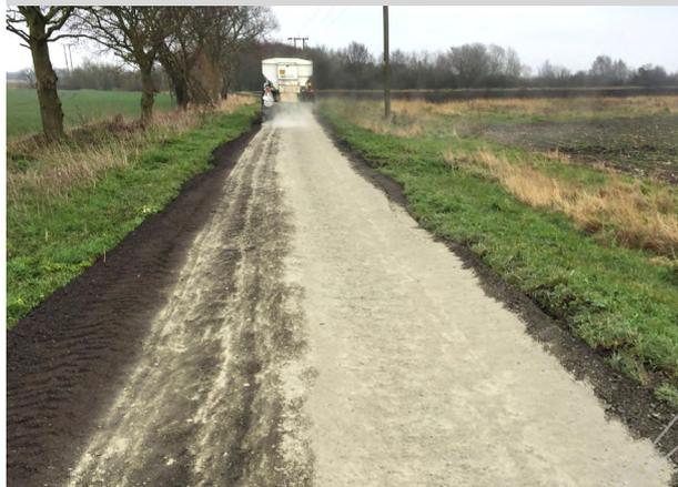
A blended cement based powder (CEM 2) was spread over the graded material placed in 2 x 1.5m widths at a rate of 6.3kg per m<sup>2</sup> (or 2%) as per the proposed design.
