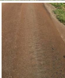
K140 Bitumen emulsion was applied to the compacted HBM so as to retain the moisture within the layer and ensure consistent curing as well as preventing the surface drying out too quickly. A protective grit was then applied to allow for trafficking prior to surfacing works. Line marking denotes the extent of the original structure of 3m width.
