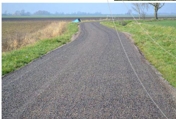
Shortly after the construction layers were complete and following a sweep of the protective grit, the HBM was Surface Dressed using a 12 and 6mm double dressing of stone and a polymer modified bitumen.
