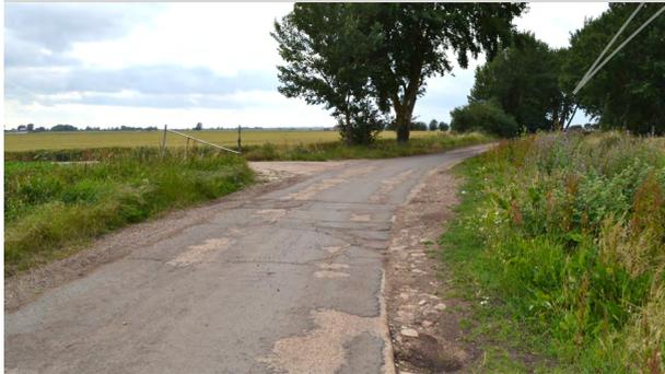
This rural road was constructed decades ago using concrete due to the peat and clay sub-grade below. The concrete had been overlaid historically with layers of asphalt which was worn and reflects deeper cracking and movement within the structure, rendering the road unsuitable for some vehicles. Level changes between slabs at joints and cracks were, in places, up to 100mm.
