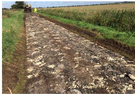
Following previous trialling of the process, Antigo were deployed with their specialist multi headed breaker to seat and rubblise the existing materials:
