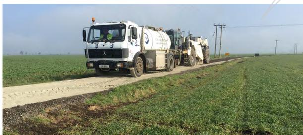
Mixing of the CEM 2 and imported planings was carried out using a Wirtgen 2000 recycling machine, adding water to achieve optimum moisture – typically 6%. Again this mixed Hydraulically Bound Material was graded and compacted to required falls.
