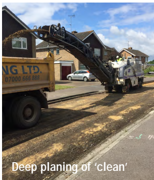
Upper coal tar layer planed off and held in lorries on site
