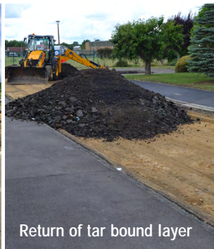
Upper coal tar layer planed off and held in lorries on site
